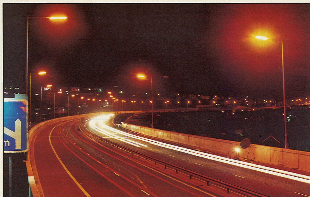
180W SOX lamps used to light 15 miles of the M5 motorway before it was widened.
